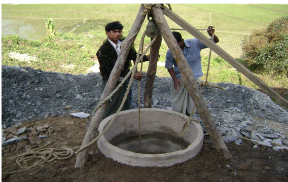
Ring well construction
