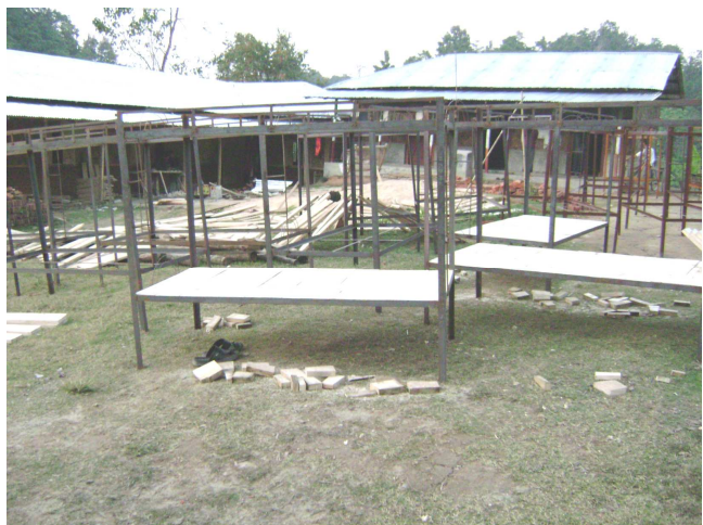
Construction of 2 storied beds
