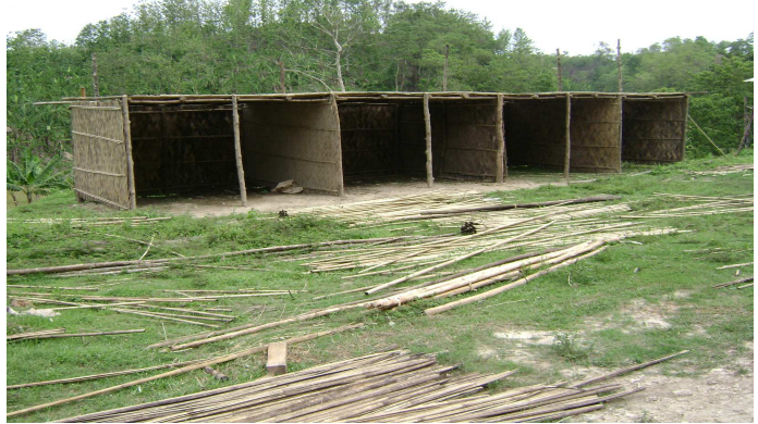
Under Construction Of Junior High school
